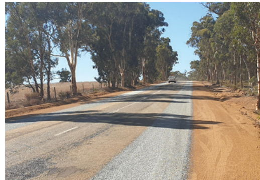
Completed shoulder widening and sealing
