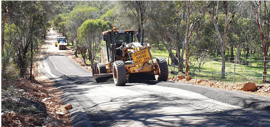
Morangup Road re-sheeting
