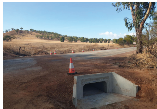
Completed culvert crossing and headwall.
