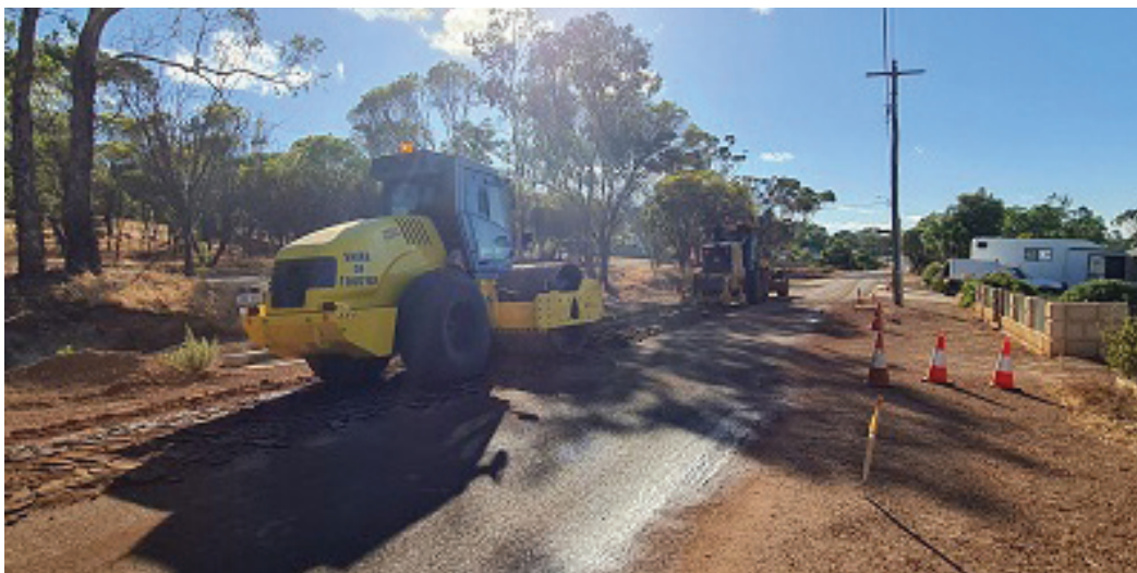
Toodyay Street upgrade – Ripping of existing asphalt
