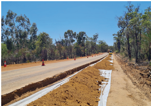
Toodyay Bindi-Bindi Road – Geotextile for soil stabilisation
