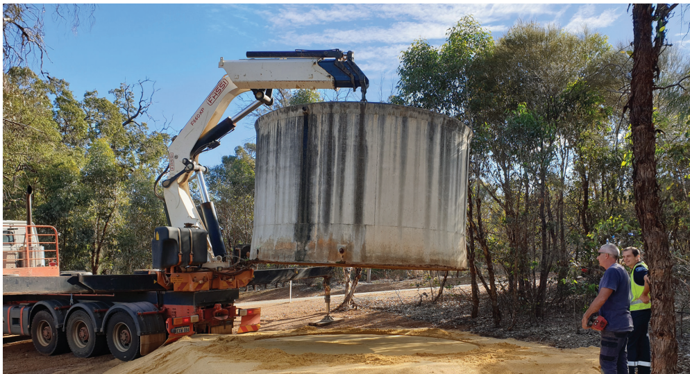
Relocating a fire emergency water tank from the decommissioned Coondle Fire Shed to Darwinia Road
