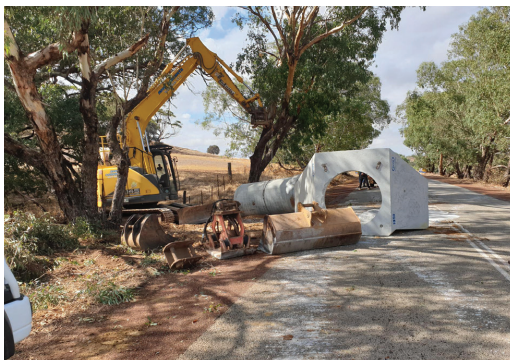
Toodyay Bindi Bindi Road – Extension of existing pipes
